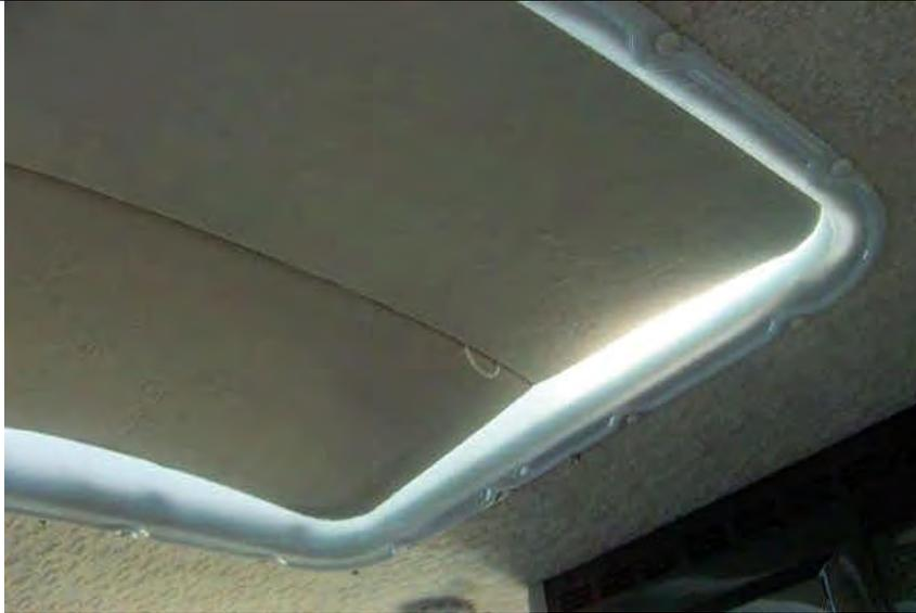
This folding insert fits snugly in the ceiling skylight bubble to control heat from the sun in summer and heat loss in the winter. It also does a good job of limiting the light that comes inside.
