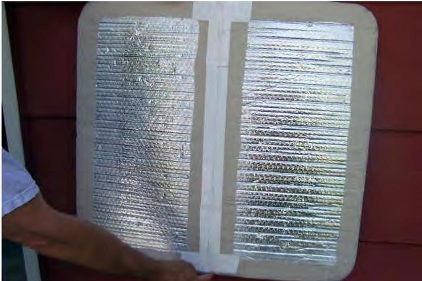
This is the Reflectix side that the sun sees. Notice that all edges of the fabric have been brought around the edges, and bonded to the Reflectix. Where the two panels butt together at the center, a 2" wide piece of duct tape serves as a hinge to fold the two panels so they may be stored easily.
