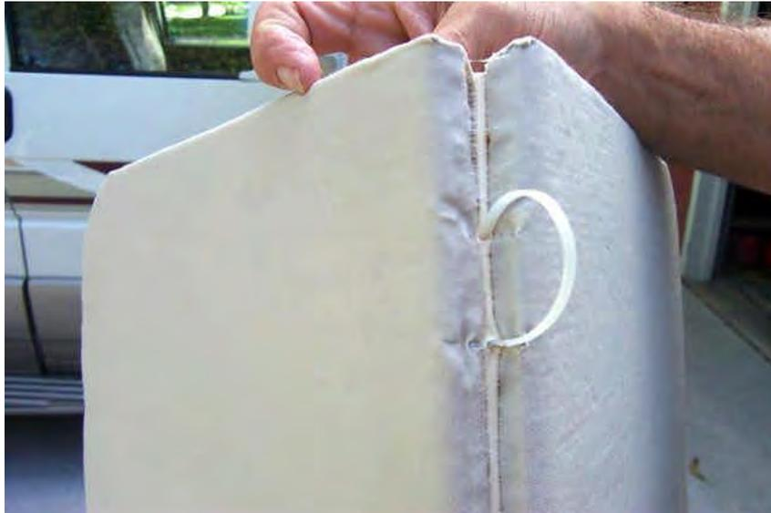
Here you can see the duct tape hinge and also the plastic tie straps, which are really needed to be able to easily remove the panels from the Skylight. Once positioned and adjusted to the loop size you want, the plastic tie straps are simply covered with duck tape to secure them in position on the top surface of the center hinge strip of duck tape. By leaving the long ends [not cutting them off] and taping the whole thing down, you may reduce the size of the loop later, if you so desire.
